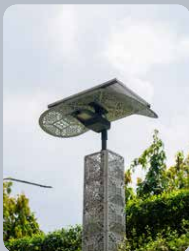
Figure 12. Street lighting with solar PV technology
